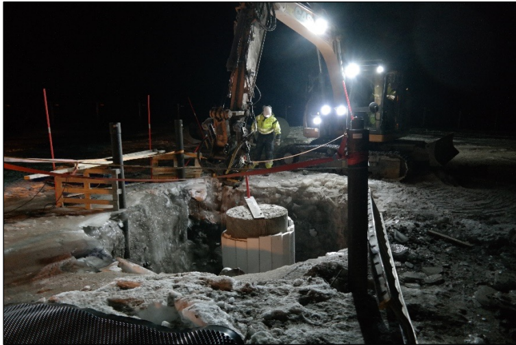
2014: Casting SLR concrete pier.
