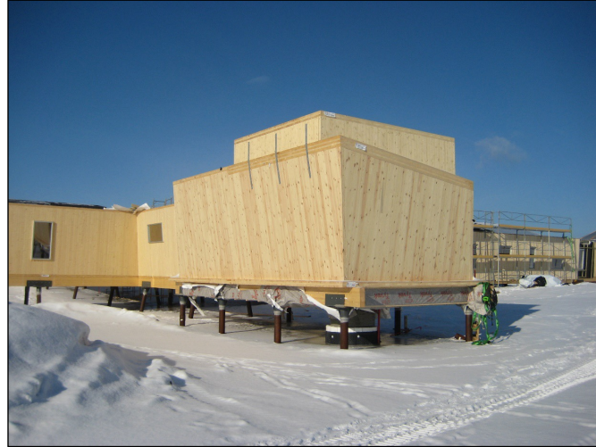
2015: SLR building construction.
